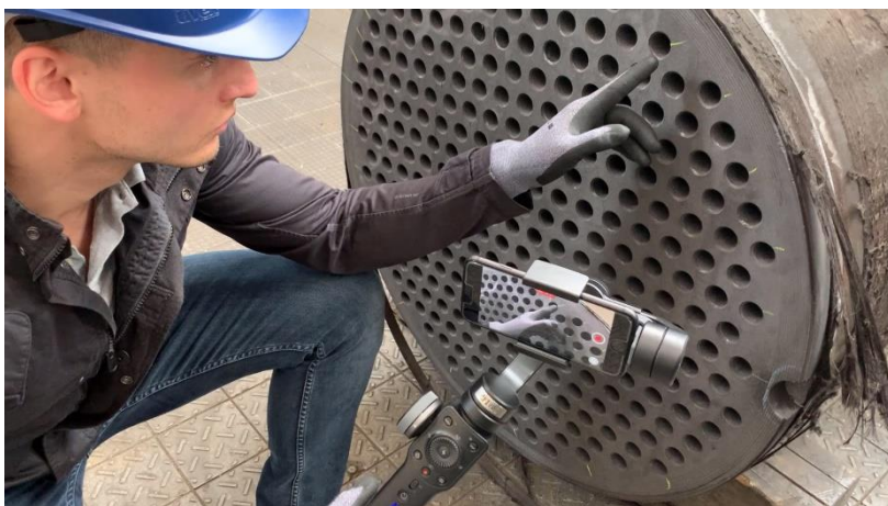
Remote Expert Service at a HCl absorber unit
