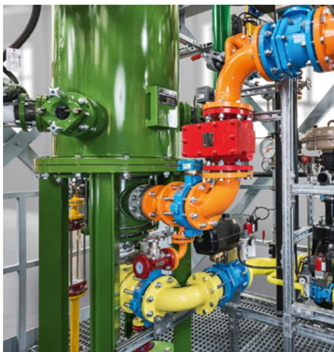
↑ Bottom-burner combustion chamber and ignition system
