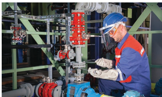
↑ Installation of DIABON® graphite pump
